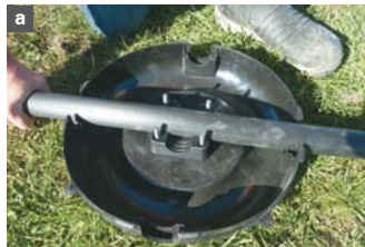
Lay pipe over Skid Base and secure in position with Cross Tee Anchor.
