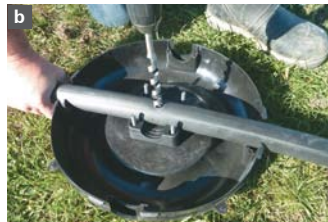
Drill 15mm (9/16") hole at required spacing for the sprinkler type being used and remove all drilling swarf. Ensure the hole is drilled perpendicular to the Pod Base.
