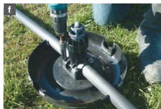
Fit O-ring seal to Pop-up Tapping Saddle Top, locate spigot into hole in pipe and fasten to Cross Tee Anchor, ensure fastening nuts are tightened evenly.
