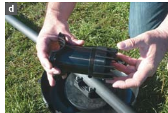
Place Pop-up Screw Cap Seal on top of Pop-up Tapping Saddle Top and secure Pop-up Screw Cap into place.
