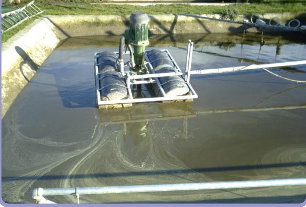
3. Primary Sump and Pump System
