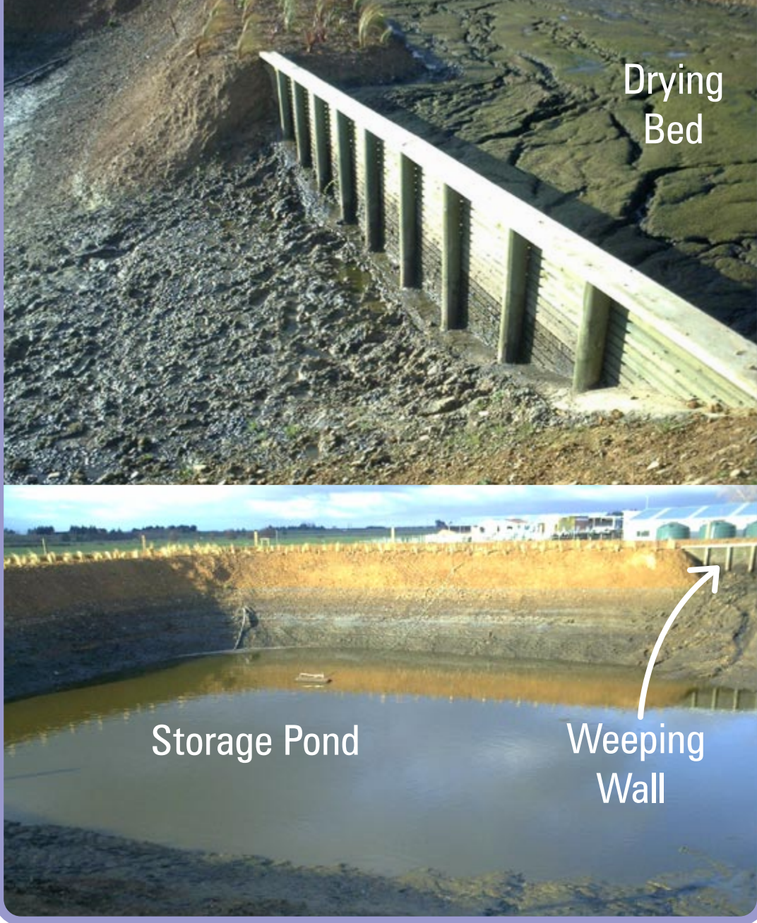
4. Weeping Wall Drying Bed & Storage Pond
